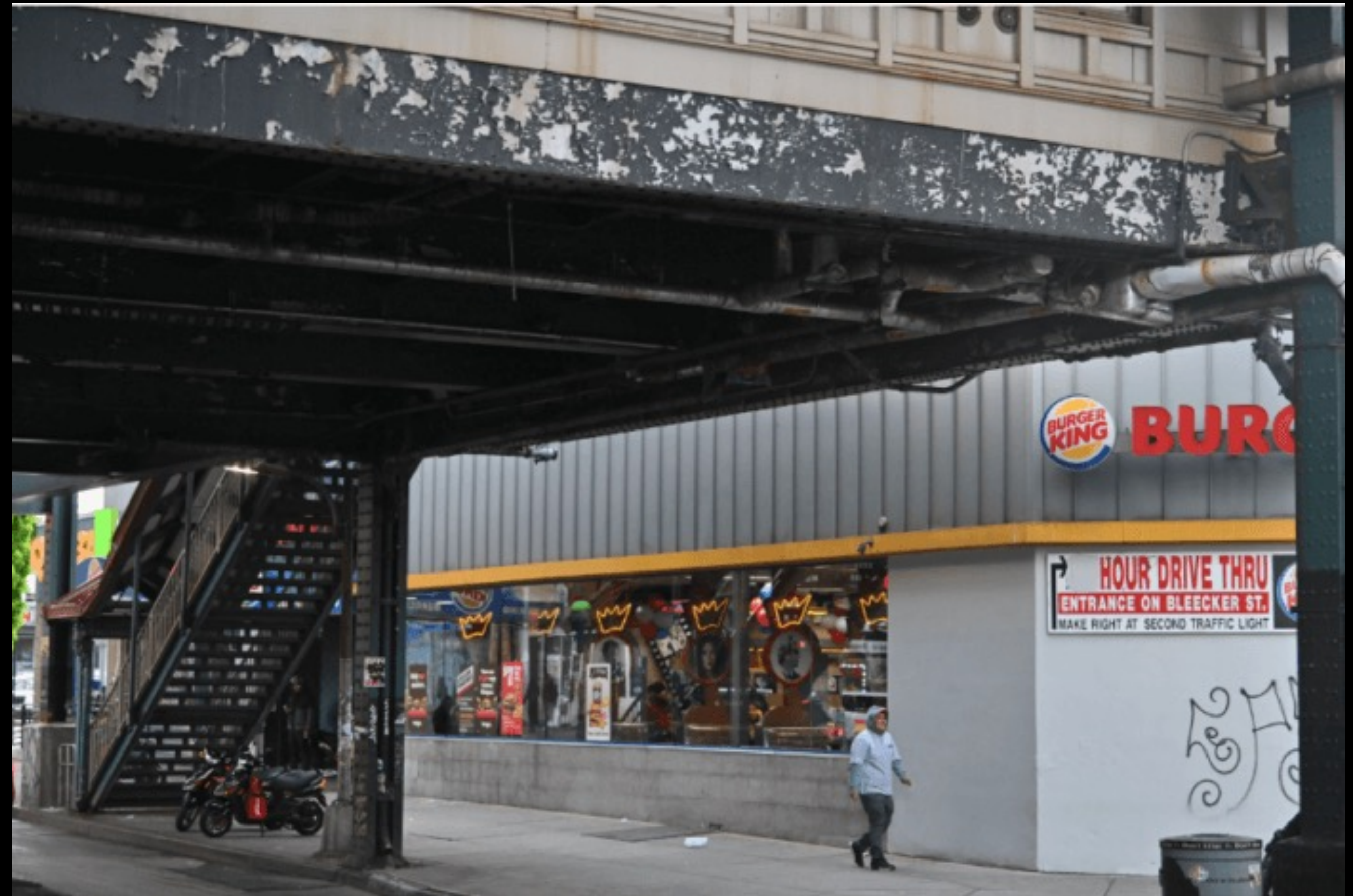
Chipping lead paint
