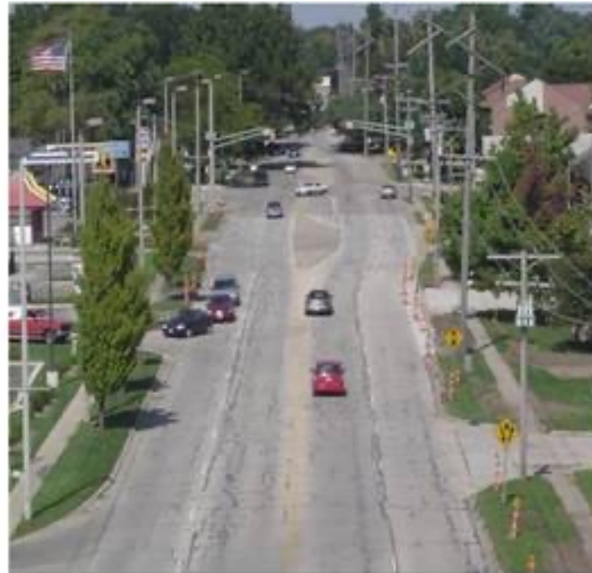
Four Lanes w/o center turn lanes
