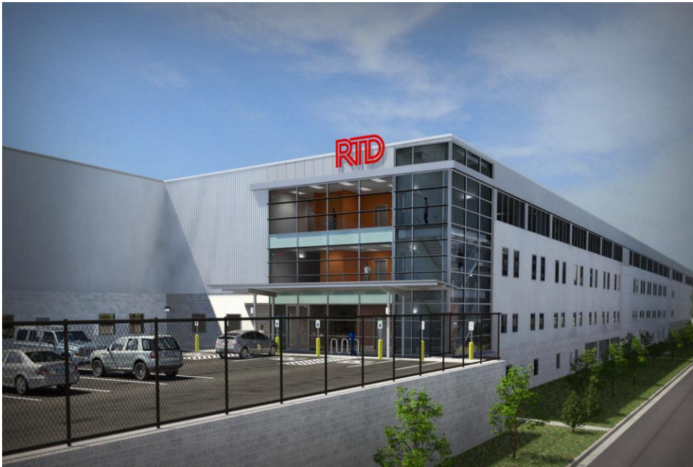
Commuter Rail Maintenance Facility
