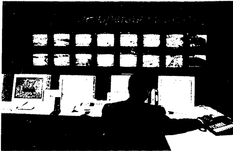
Traffic Operations Center. Supervisors and state-of-the-art computers monitor traffic conditions via 35 TV cameras and hundreds of in-pavement sensors.
