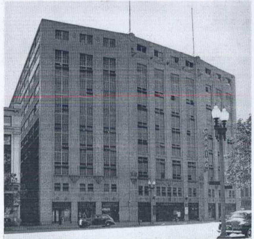
PLATE V.—The simplest and most elaborate forms of off-street parking structures. The structure above is little more than a parking lot in several levels. The lower structure is a multi-storied garage in which vehicles are parked and service rendered by a staff of attendants and mechanics.
