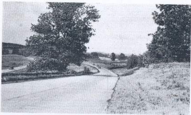
This view of the Eastern State Parkway near Fishkill, New York, typifies approximately the kind of construction proposed for rural sections carrying upwards of 3,000 vehicles a day. Note that the opposing traffic lanes are constructed as practically separate roadways on different grades, each fitted to the topography with resulting reduction of cost. Such sections of the system may be built at costs of from $100,000 to $150,000 per mile, depending largely upon the costs of right-of-way and grade-separating structures.
