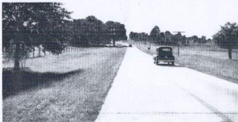
Sections of the system designed for traffic of volumes between 1,000 and 2,000 vehicles per day should be similar in most respects to those serving smaller traffic volumes, but surfaced with pavements of higher type. Cost may range between 30 and 70 thousand dollars with variations in grading quantities and number of grade-separated intersections. The Alabama highway pictured above conforms approximately to the standards proposed.
