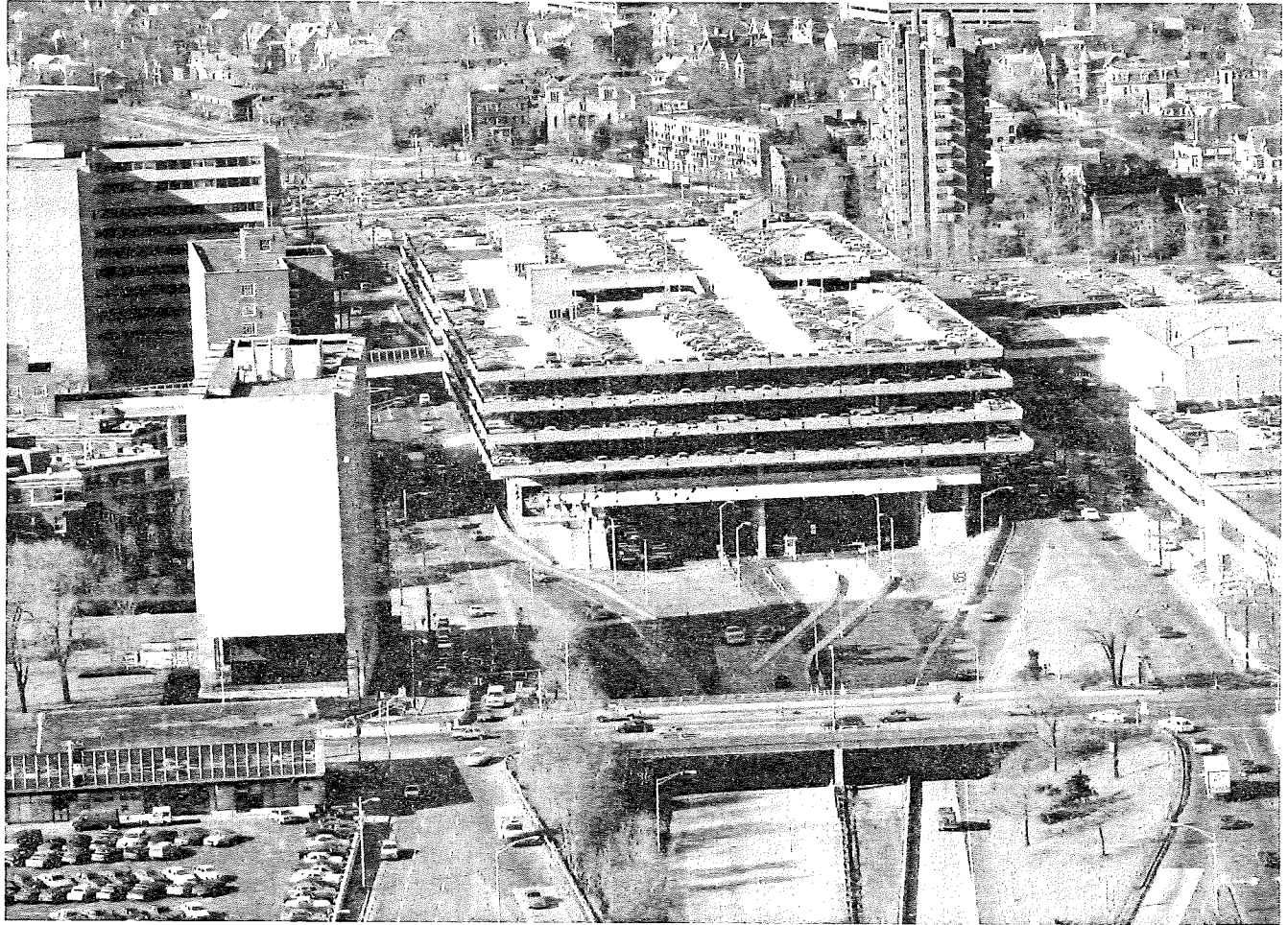
Figure 7.2. New Haven, Connecticut's 2,800-space Air Rights Garage
