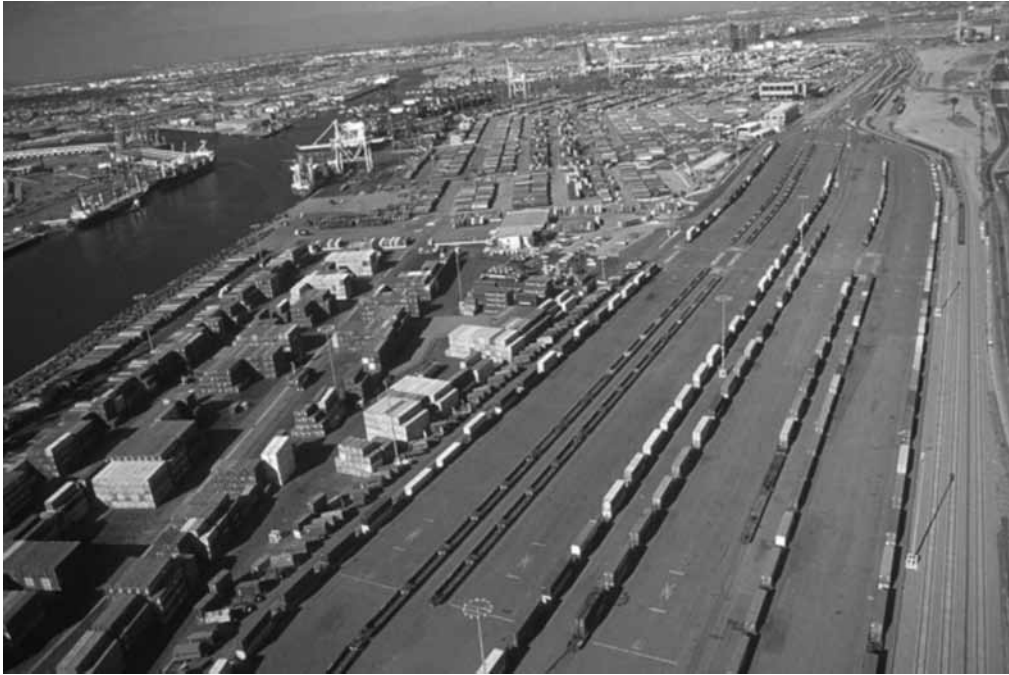
► Figure 11-9 Port of Los Angeles
