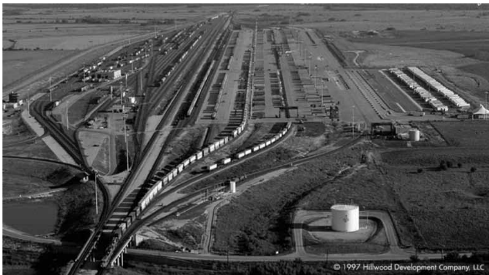
► Figure 11-8 BNSF Railway's Alliance Intermodal Facility, Fort Worth, Texas
