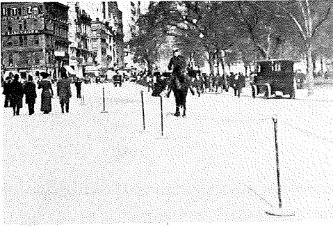
The roping system recommended by Mr. Eno for Union Square was widely copied as an inexpensive and quick measure to control traffic.
