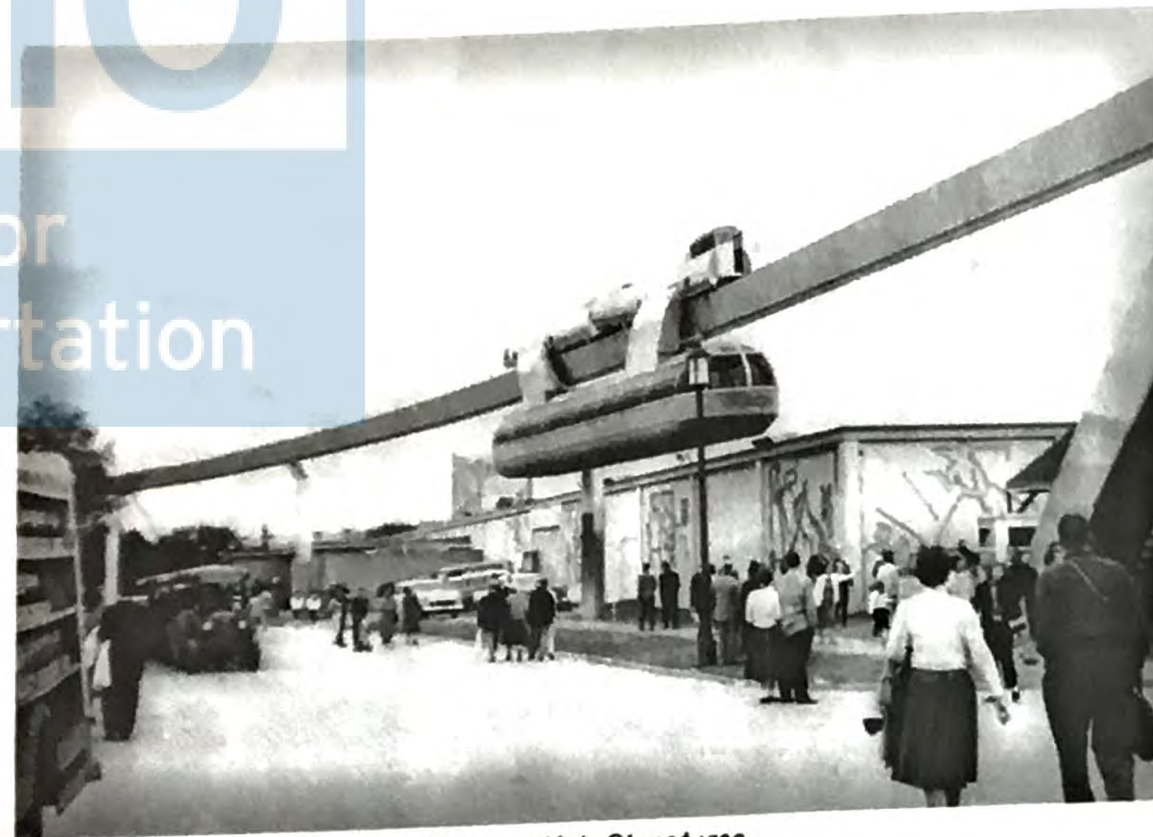
Monorail Cars Require Substantial Structures, Even for Low Speeds--Amusement Park Installation at Dallas.
