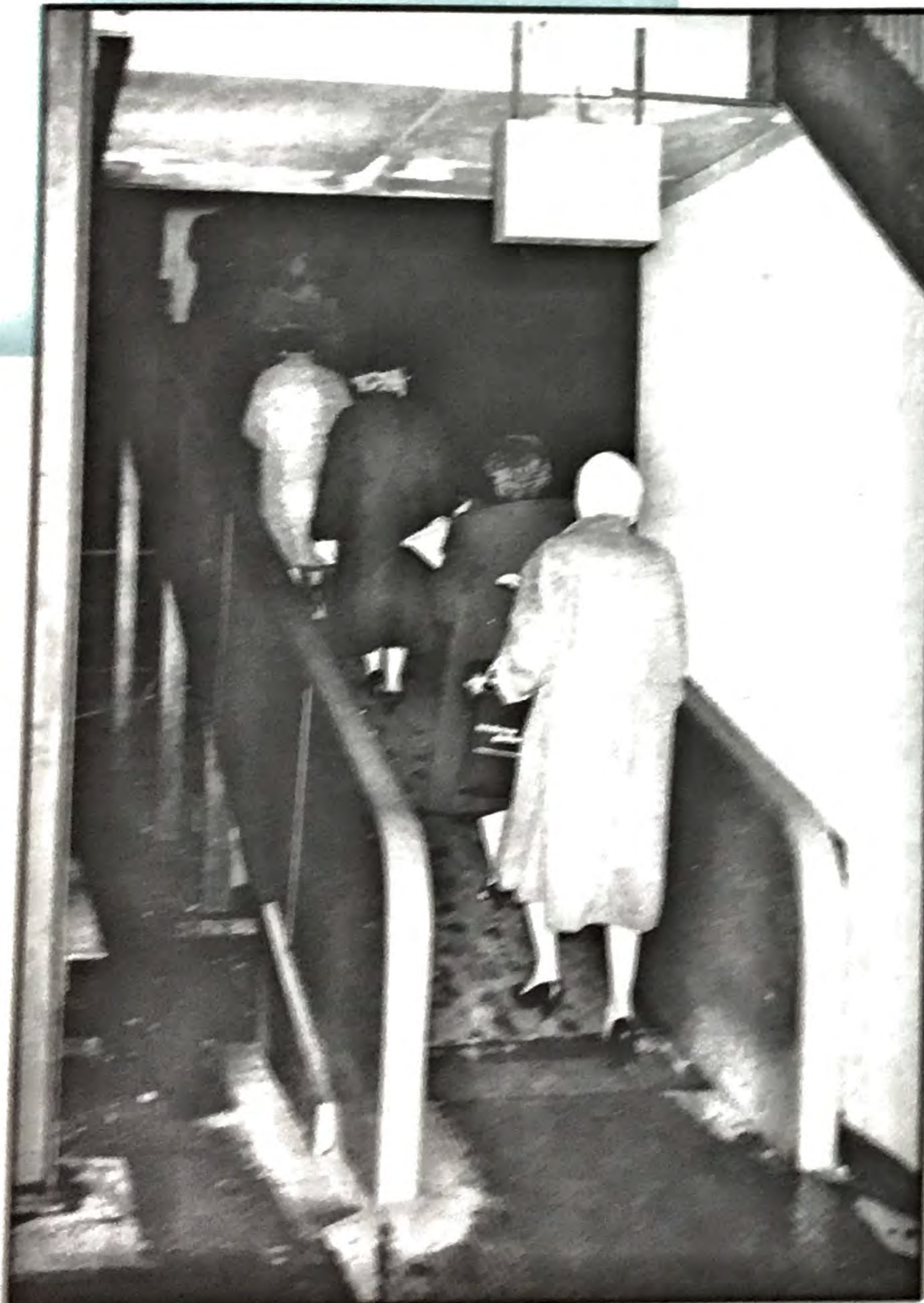
Moving Sidewalks are Especially Applicable Where Steep Ramps Would Otherwise be Required
