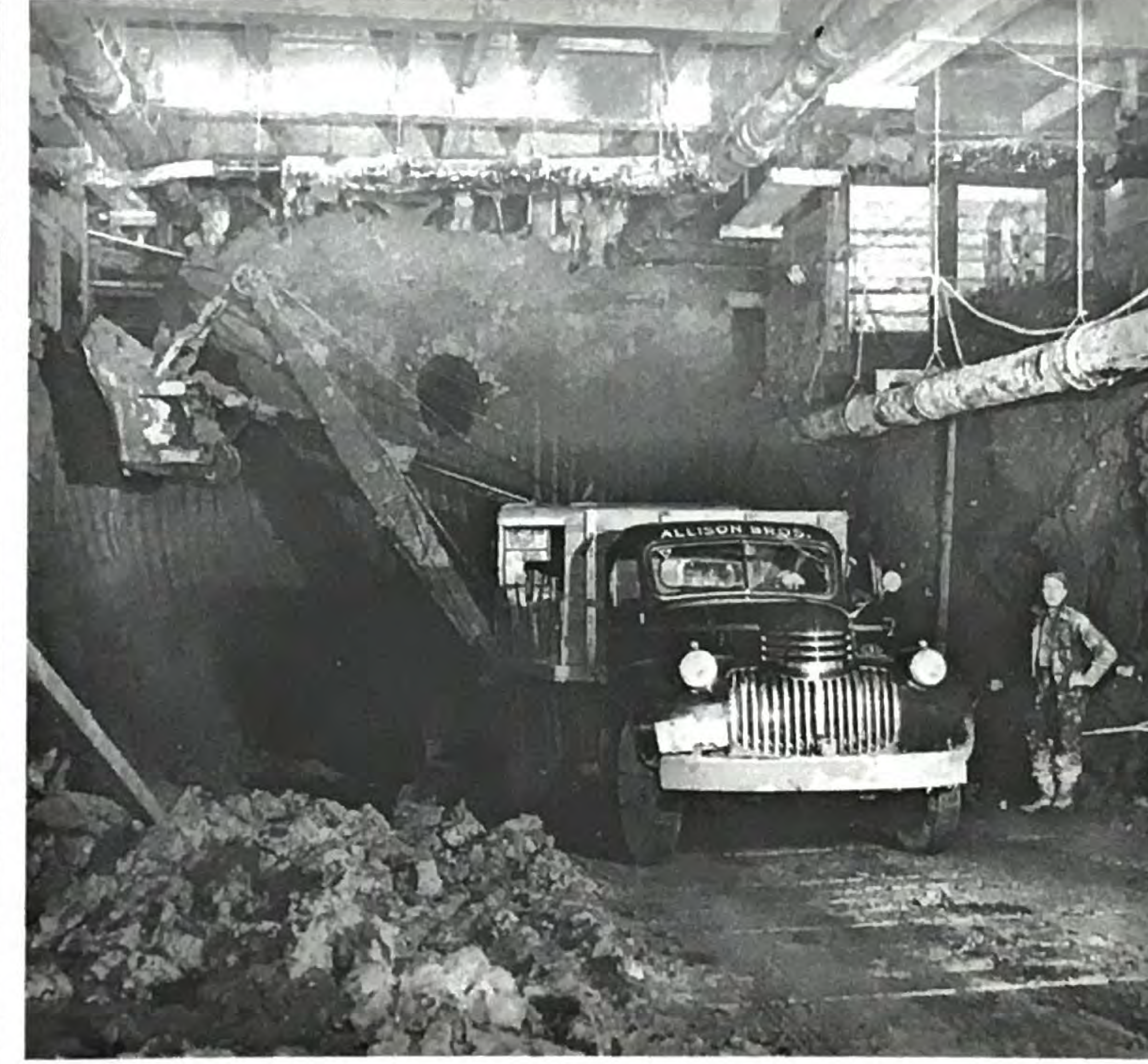
Subway Construction Proceeding Under Temporary Decking of Street Yonge Street Subway -- Toronto
