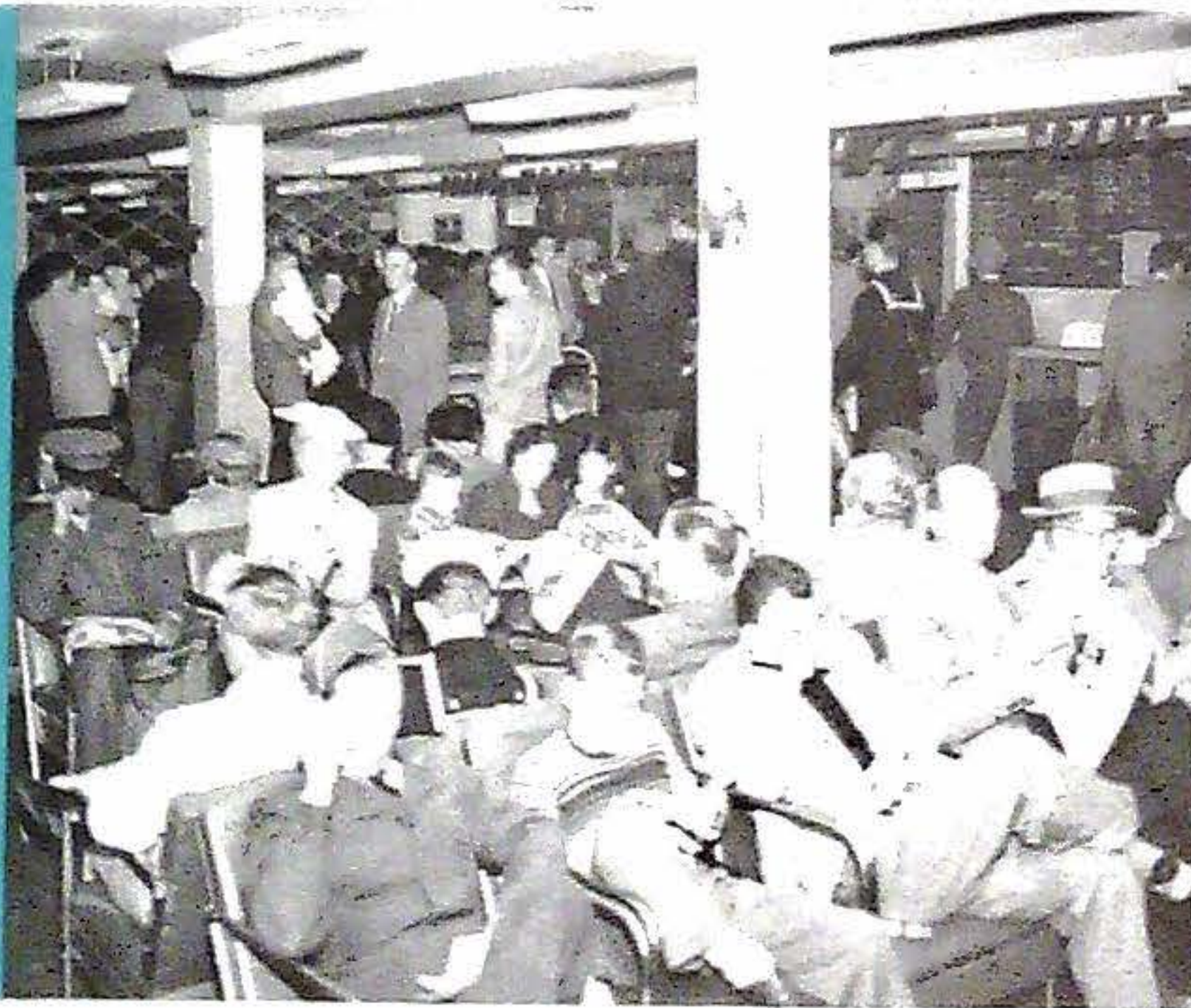
Waiting rooms are already crowded.
